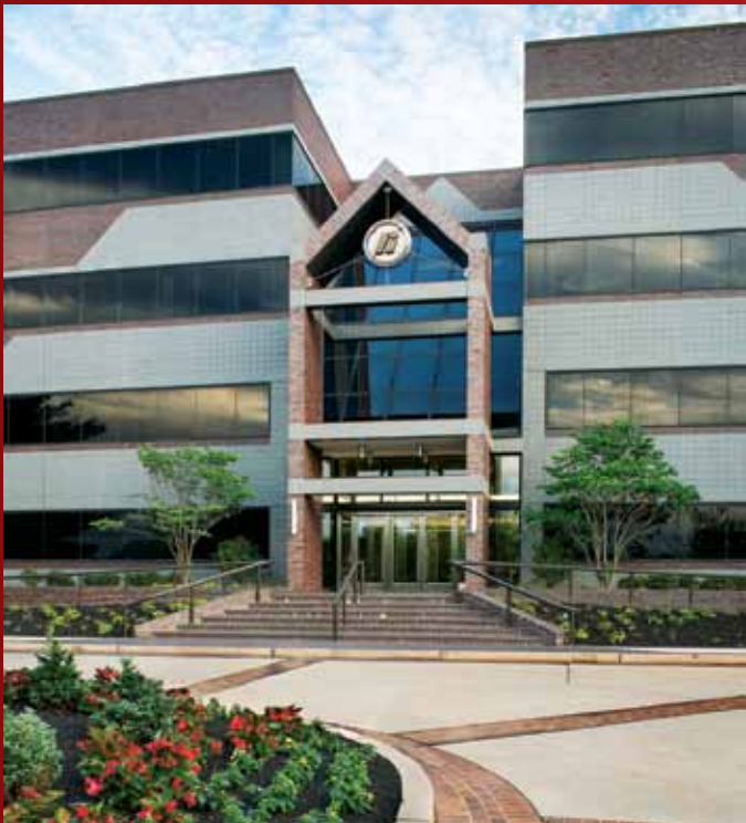
The Corporate Office of the High companies, Greenfield Corporate Center, Lancaster, Pennsylvania, has received the ENERGY STAR®.
