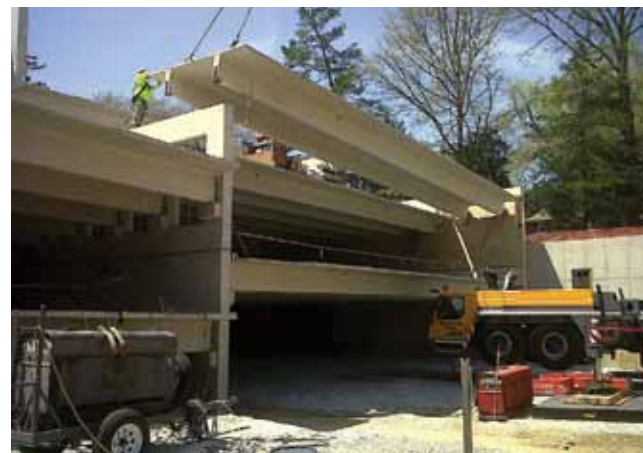
Top: High Structural Erectors erected over 16,000 tons of structural steel for the Maryland Transportation Authority's $208 million I-95 / I-695 Interchange, Phase 1 project in Baltimore County, Maryland.
