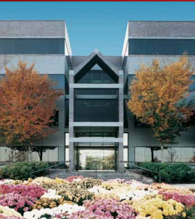
The Corporate Office of the High companies, Greenfield Corporate Center, Lancaster, Pennsylvania, has received the ENERGY STAR®.
