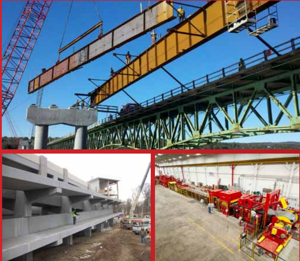
High Industries is made up of affiliated companies that serve construction and manufacturing markets. Top: A plate girder bridge is erected for the Virginia I-495 HOT Lanes project. Located in the Washington, D.C. Capital Beltway, the project totaled over 21,500 tons of steel fabricated and erected by High Steel Structures; High Transit shipped the job. Bottom Left: Cantilevers featured in the four-story, 683-space precast concrete parking garage built by High Concrete Group for the Philadelphia Zoo, in Philadelphia, Pennsylvania. Bottom Right: High Steel Service Center's HIGHSL® processing line comprises a Bradbury Group eDrive® roller leveler, a Bradbury heavy-gauge roller leveler, and a Red Bud Industries® stretcher leveler to provide panel-flat carbon steel that is 100 percent stress-free.
