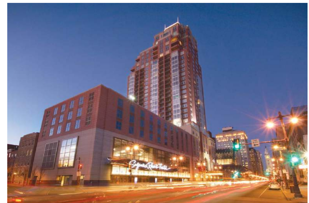
Symphony House, a luxury condominium high-rise in Philadelphia, Pennsylvania, was designed using lightweight CarbonCast architectural panels that saved superstructure costs and contributed to better interior layout.
